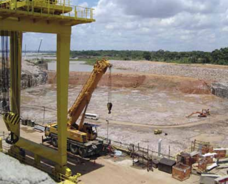
HUBER+SUHNER on site: 200 customised fiber optic systems by 2015
